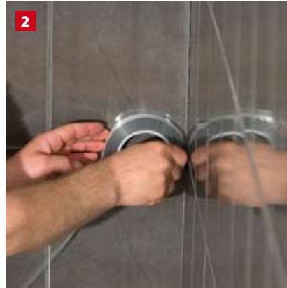
2 First fix the outside of the tape to the wall, with the fold on the tape placed right into the corner. Apply the tape down the wall while pulling off the backing paper.
