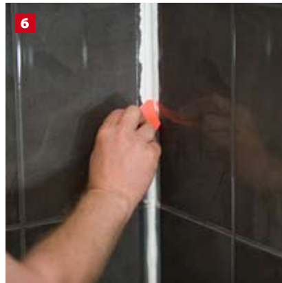
6 Smooth down the whole joint using the accompanying joint former, keeping it as perpendicular as possible to the wall.
