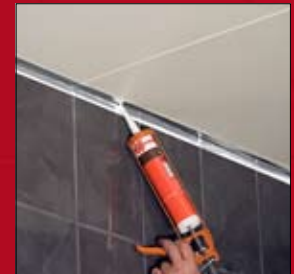
Ceiling/wall joints in bathrooms
