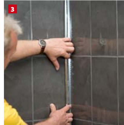
3 Unfold the inside of the tape and fix it to the wall. Make sure not to pull the tape out of the corner.
