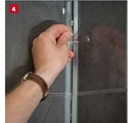
4 Remove the plastic film. Only the metal tape should be left on each side.
